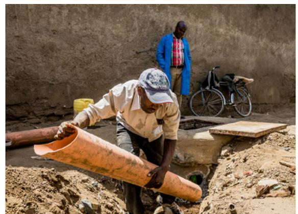
**Image:** Connecting a pipe to a trunk sewer line, Nakuru, Kenya.
