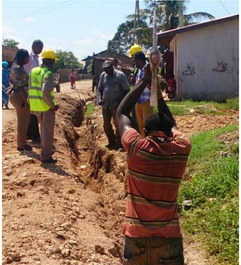
Image: Water pipeline excavation in Mombasa.
