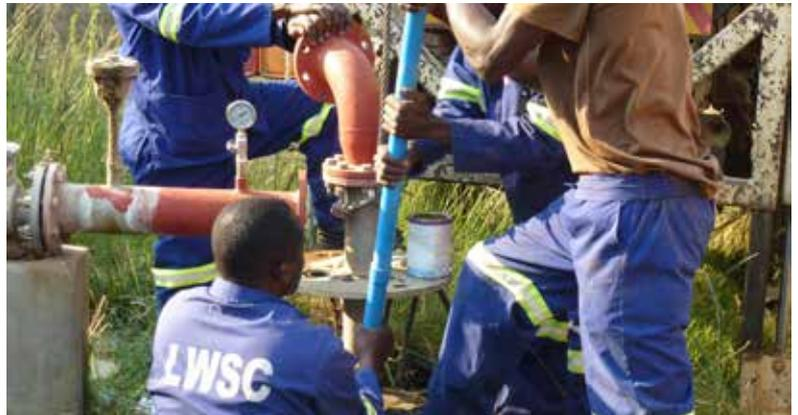
Image: LWSC installing dip tubes & data loggers
