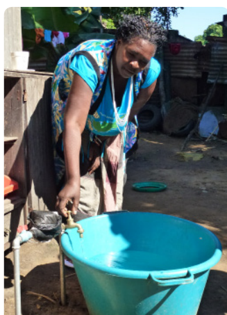
A new household water connection in Xipamanine, Maputo
