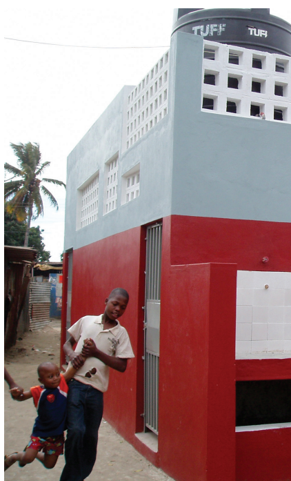
Tchemulane communal facility
