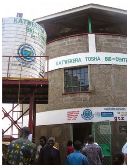
BioCentre facility in Kibera
