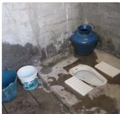
Well-maintained communal toilet in Bangalore
