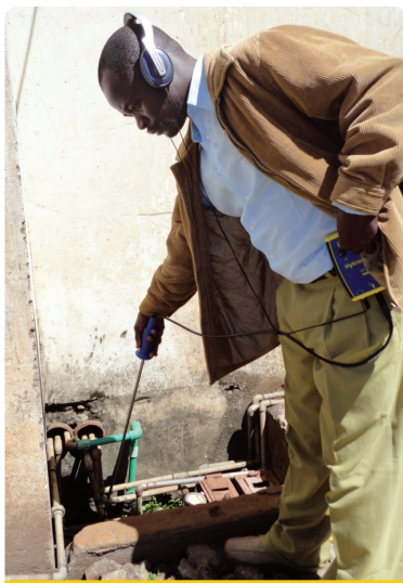
Leakage detection training in Nairobi, Kenya, where WSUP is supporting a similar NRW reduction programme.
